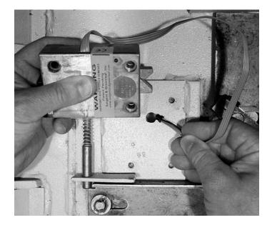
Once you've double-checked to make sure the wire cable is not crimped or in contact with any sharp surface, attach the lock to the safe's mounting plate. Use the three  $1/_4$ -20 or M6 (metric) mounting screws provided. Tighten securely so the lock is attached firmly to the plate.
