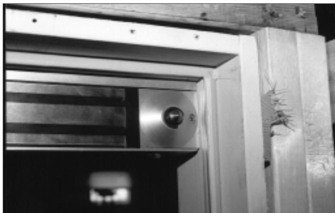
7. The locator pin is inserted and ready for marking the door.
