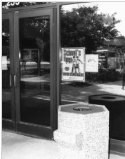
2. To handle the weight and abuse this door receives, a continuous hinge is applied.
