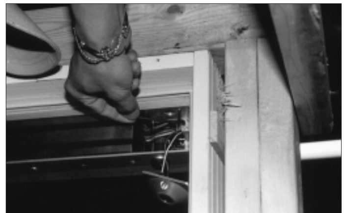
3. Attach the DynaLock to the T-track.
