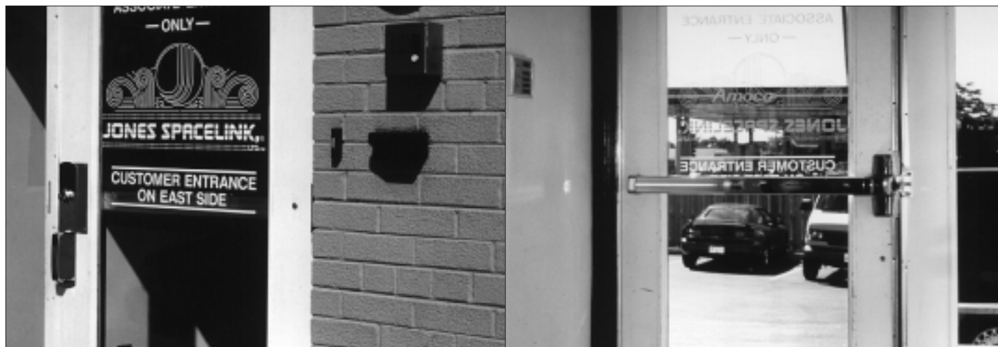
1. For this application, a Von Duprin 99 ELR is used.
