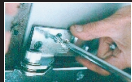
7. Attaching the lower pivot hinge.
