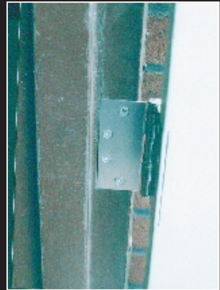
6. With hinges attached, mount the door to the frame.
