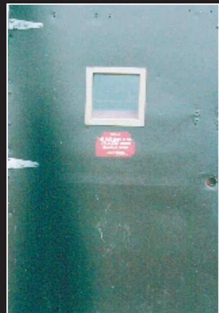
1. The nice new door is now held in place with strap hinges.
