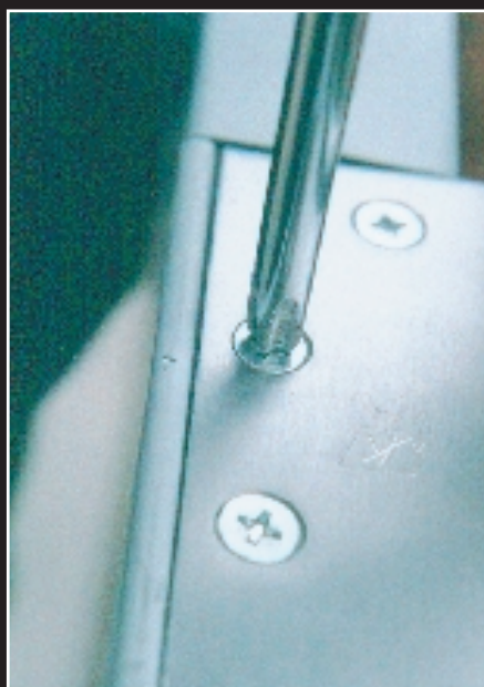
5. Attaching the new hinges.
