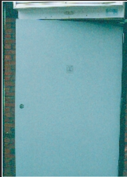
8. The door is up and ready for the rest of the hardware.
