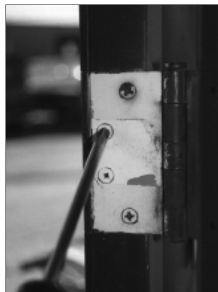
2. Use the correct tool for removing the hinge. In most instances a #3 Phillips screw driver is used.
