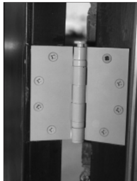
5. The installed hinge. Notice that the hinge pin removes from the top. This is the correct direction for installing a hinge.
