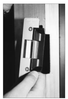
12. After checking for the initial fit, the U-Tabs were installed and the strike mounted to the frame.
