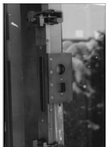
5. After removing the existing push bar and pull handle, the HIT-45 is clamped to the door and ready for cutting.
