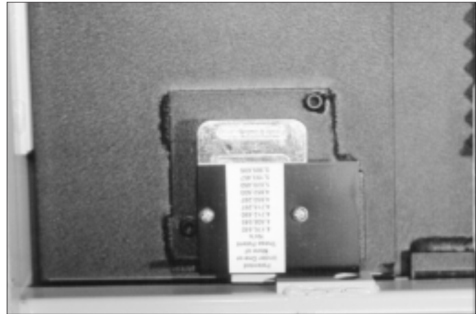
6. Rear view of sliding door with relock cover in place. Cover is held on by combination lock cover screws.
