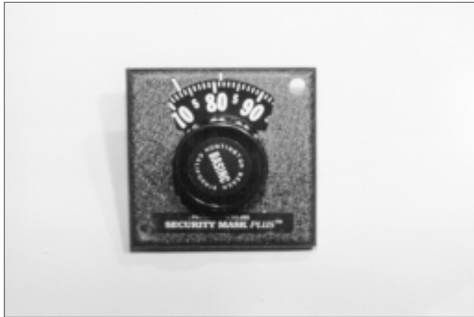
5. Security Mask and Dial. Note two holes drilled in upper right and lower left corners of cover.
