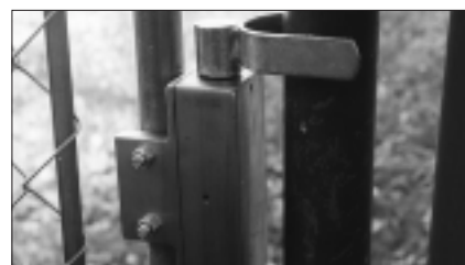
19. The completed installation.
