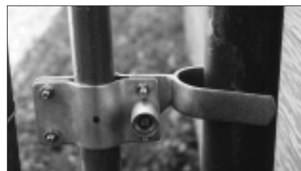
5. The installed Push Button lock.
