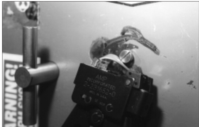
6. Using the AMP tool to connect the 8-pin connector to digital lock.
