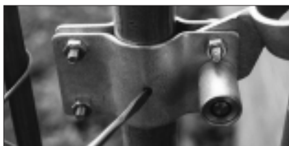
4. Tighten the set screws on the sides of the collars.
