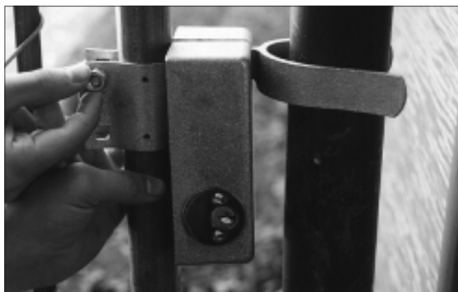
12. Holding the unit up to the gate, install the carriage bolts.
