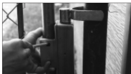
17. Marking the mounting hole for drilling.
