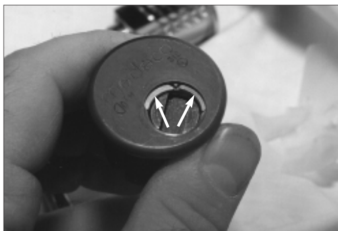
5. The steel inserts on this mortise cylinder also prevent easy drilling.
