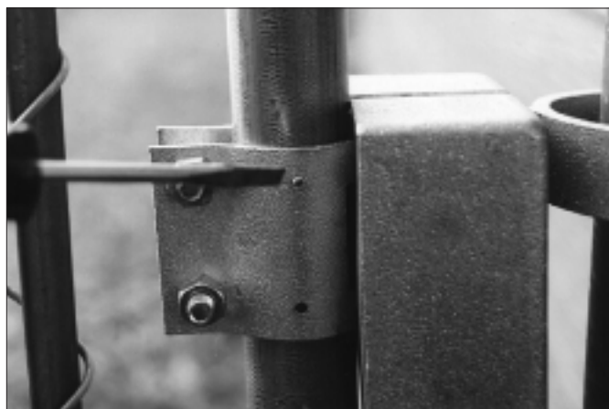
13. Tighten the set screws on the collar.
