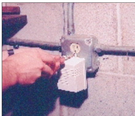
10. Plug in the line carrier transformer into an unobtrusive plug that is not controlled by a switch.
