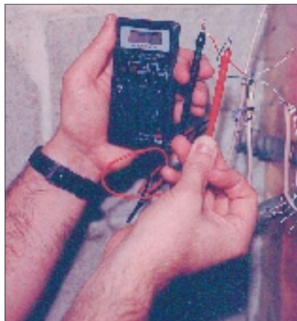
5. Use the voltmeter to determine which lines are Telco lines and which are premises phone lines. The 41.7 volt reading indicates the Telco line; the 136 millivolt (a fraction of a volt) reading indicates the premises phone line.
