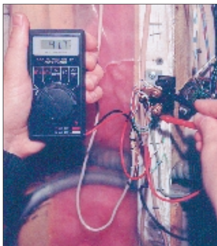
3. The digital voltmeter indicates which Telco terminal is positive and which is negative. This 41.7-volt reading indicates that the bottom terminal (touched by the red lead) is positive. The -41.7 reading indicates that the red lead is touching the negative terminal.
