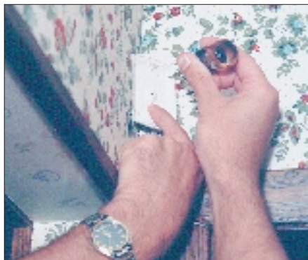
11. Sensors come with a variety of mounting brackets. This is a corner-mounting bracket for a wireless PIR motion sensor.
